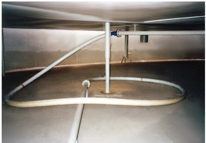
Installed Drain Pipe System
